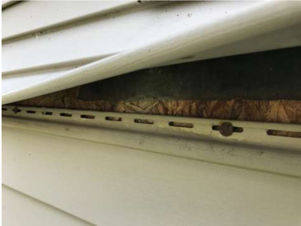
Building 3 - 26 Courtyard. Sheathing stained and flaking under 2 nd floor window.
