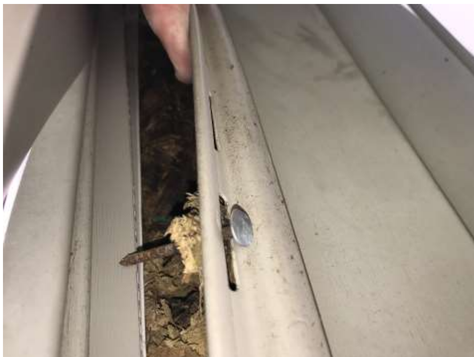
Building 1 - 1324 North West Street. Rot under window.
