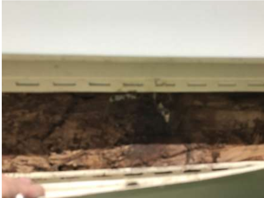
Building 6 - 60 Courtyard. Sheathing rotted under window.
