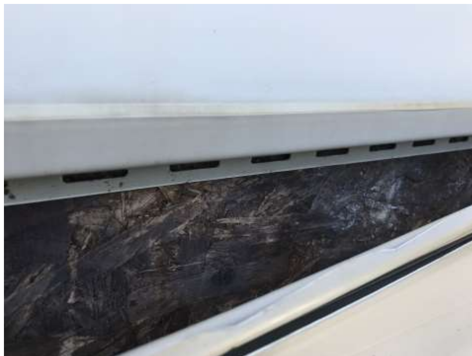
Building 1 - 2 Courtyard Drive. Rot under window.
