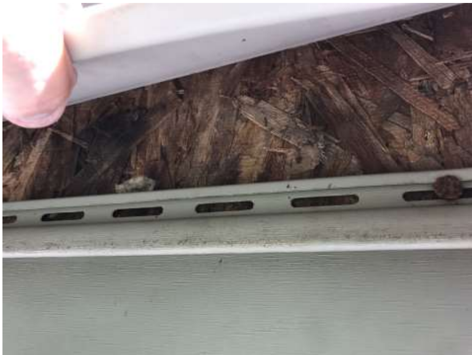
Building 1 - 1324 North West Street. Rot under window.
