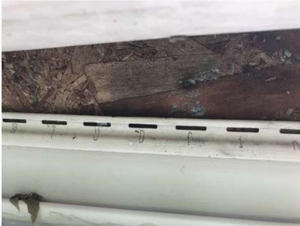
Building 6 - 66 Courtyard. Water stains, mold and ants observed.
